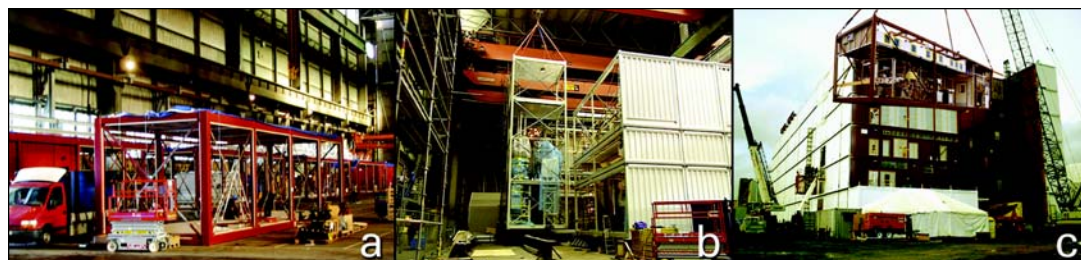
Figure 1. Innovation of focus: modular facility technology. a. Facility modules fabricated in a factory; b. An entire facility assembled and pre-tested in a factory; and c. Facility modules rapidly assembled at site.
