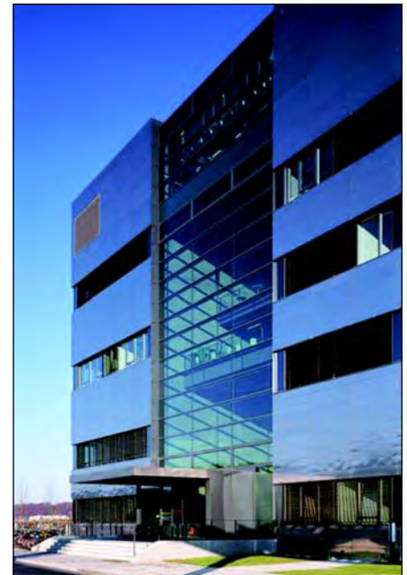
Main entrance of the pharmaceutical R&D building.
