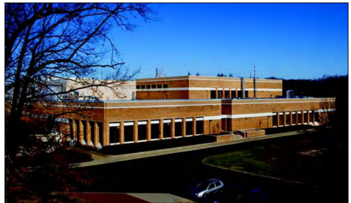
BMS CSO/DPTC facility.
