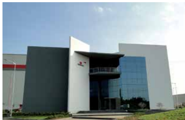
Front view of administrative block
